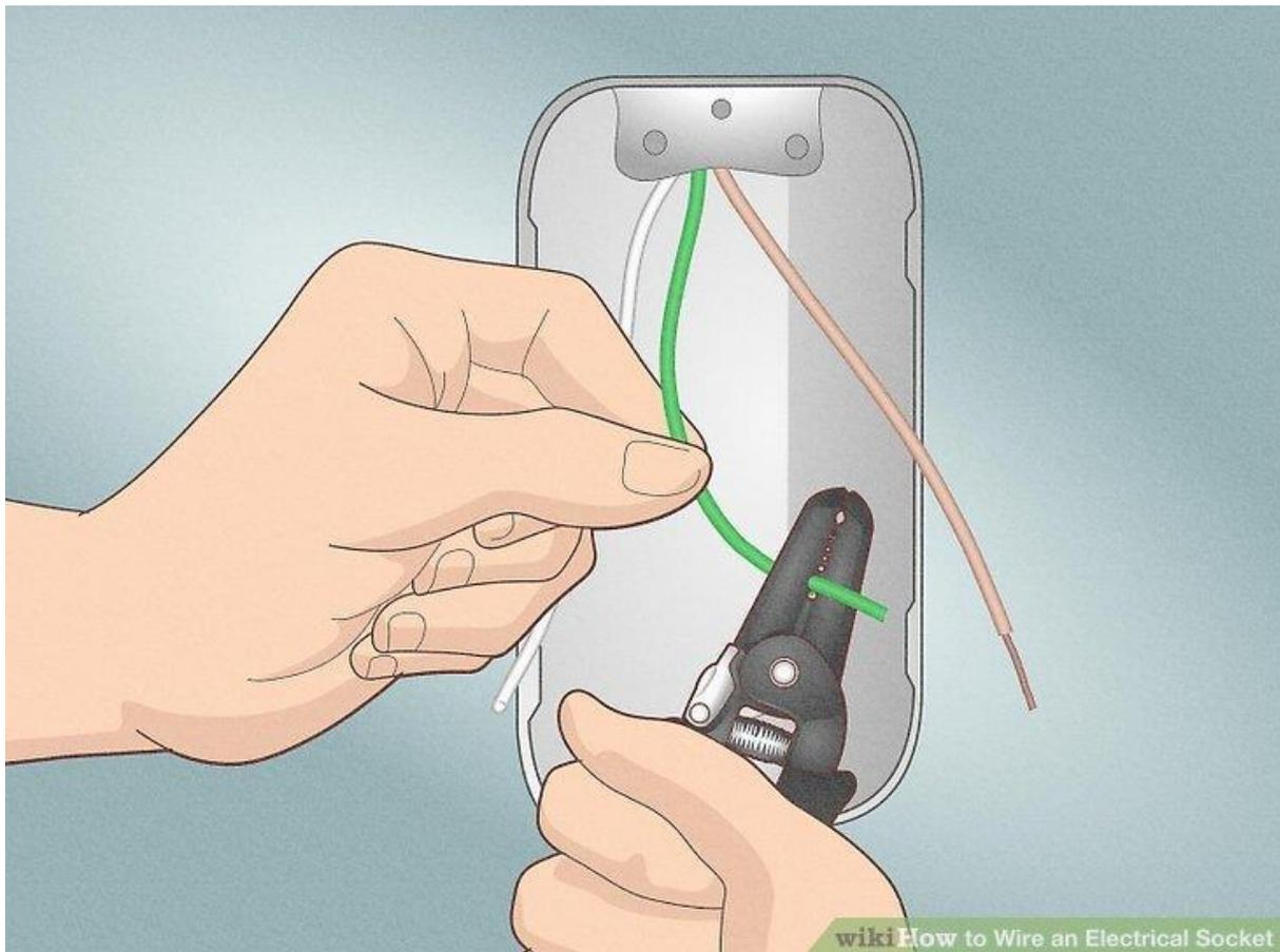
**Strip the ends of your wires.** If the wires are frayed or nicked, cut the damage off, then strip off roughly  $\frac{3}{4}$ " (2cm) of insulation. You can do this [using a wire stripper](#) or [a utility knife](#). Take care to avoid nicking the metal of the wire, which can cause electrical faults later.[\[13\]](#) Err on the side of under-stripping so you can correct later.
