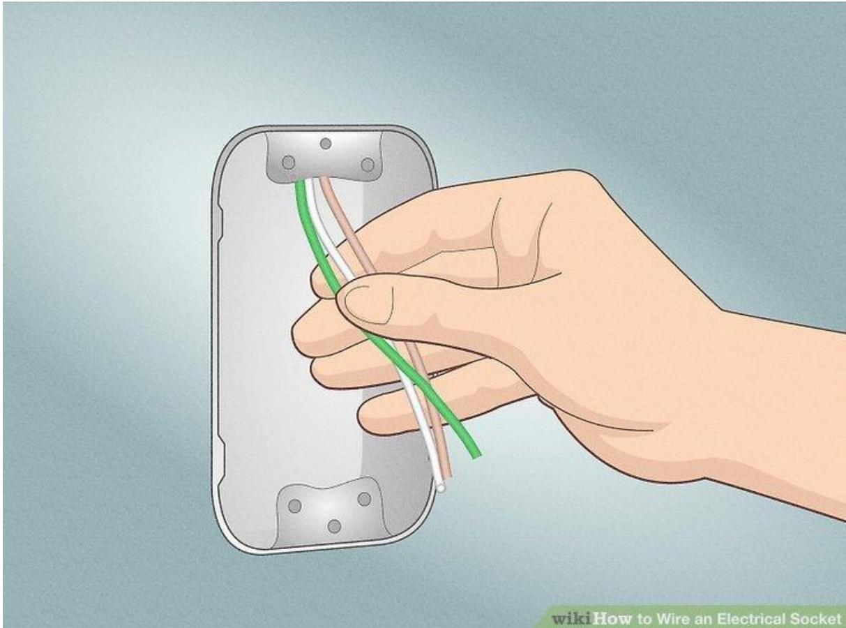
**Identify the live, neutral, and ground terminals of the socket.** A standard modern outlet for household use should have three terminals for connecting the appropriate wires.
