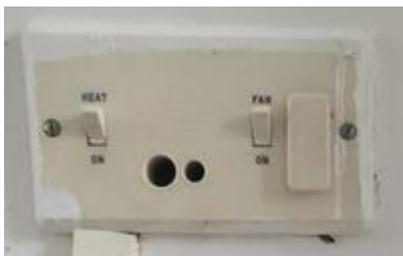
AEI Storage heater switch with separate supplies for (unfused) off-peak supply on dedicated radial circuit and (fused) boost/fan supply on the socket circuit.
