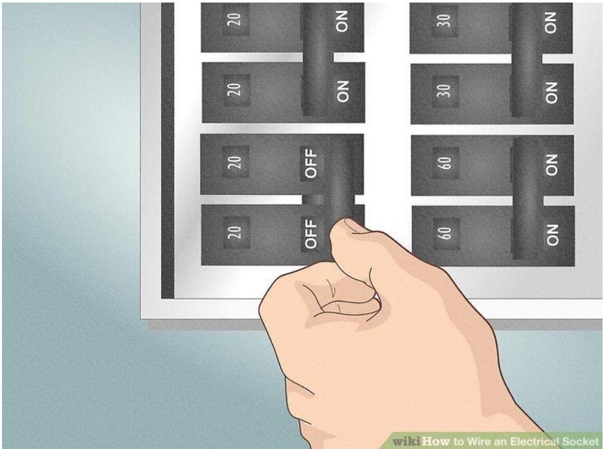
**Switch off the power.** Flip the circuit breaker or remove the fuse that powers the outlet you will be working on. If you're not 100% sure which power source to cut, turn off the power to your whole home and work with a flashlight.
