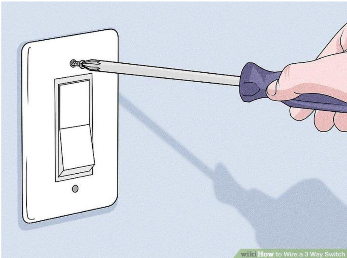
**Replace the switch box covers.** Screw the switches into the electrical box and secure the wall plate over the opening. Flip the breakers back on and test the switches.
