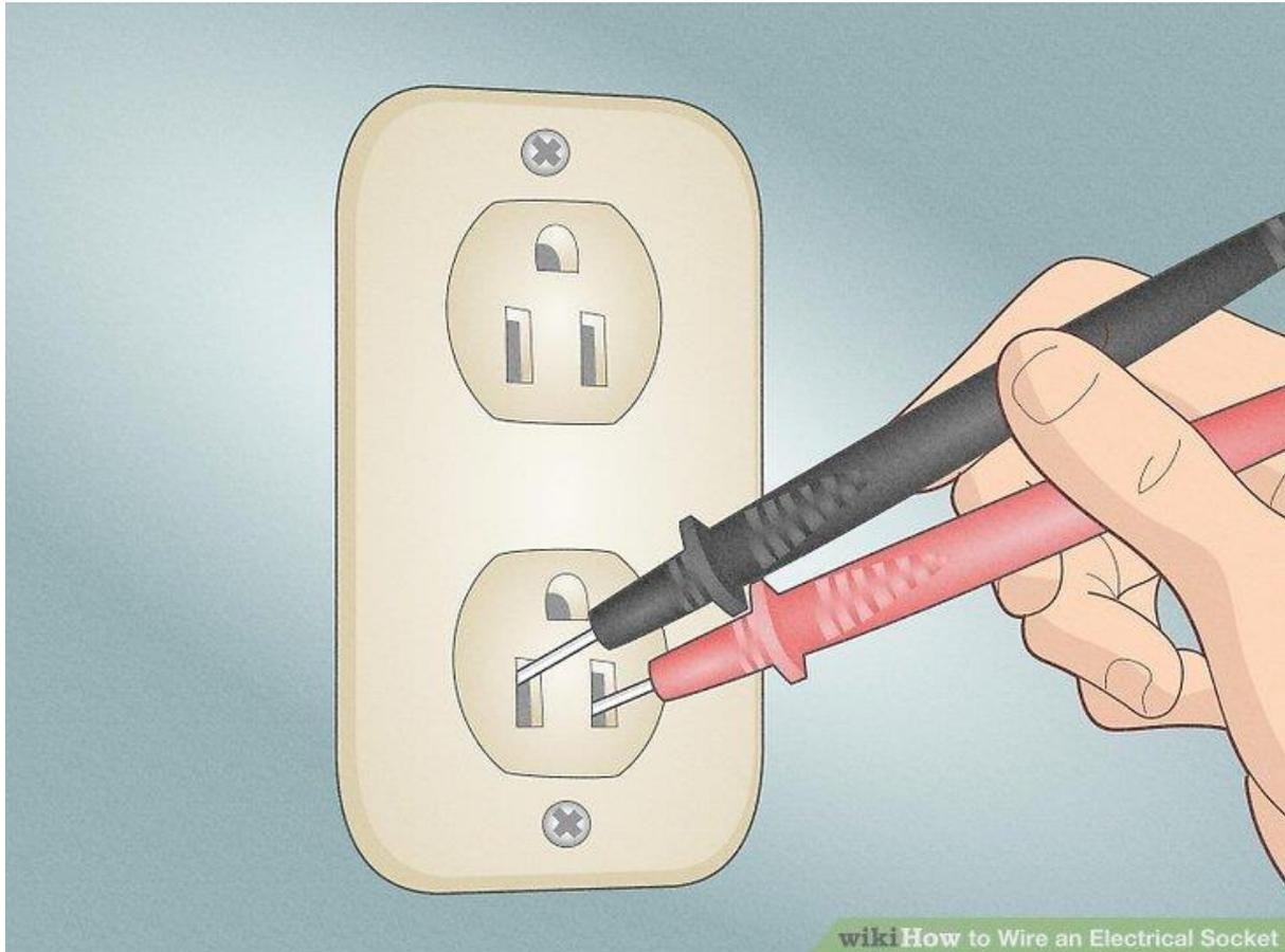
**Test the voltage.** Never assume that the wires are dead without testing. Test a live circuit first to confirm the tool is working, then test the circuit you're working on. If you get a voltage reading, the outlet is still live and cannot be worked on.
