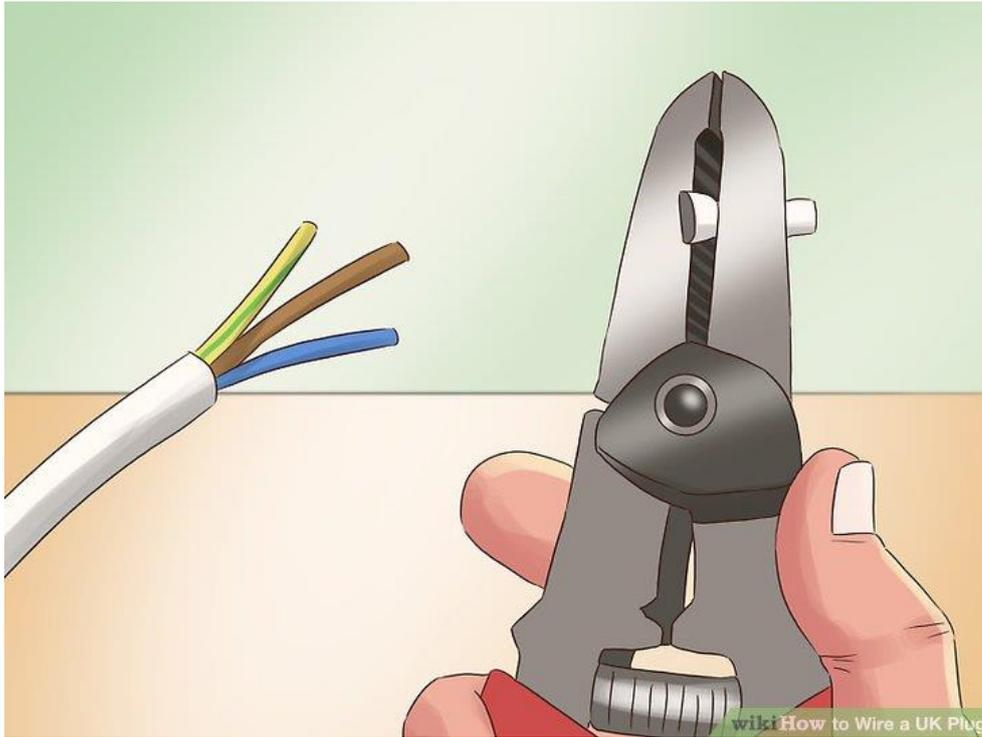
Strip the end of the thick cable coming from the appliance into the plug, using wire strippers. Take off roughly 3 centimeter (1.2 in) of white covering, leaving you with three thinner cables.[\[1\]](#)
