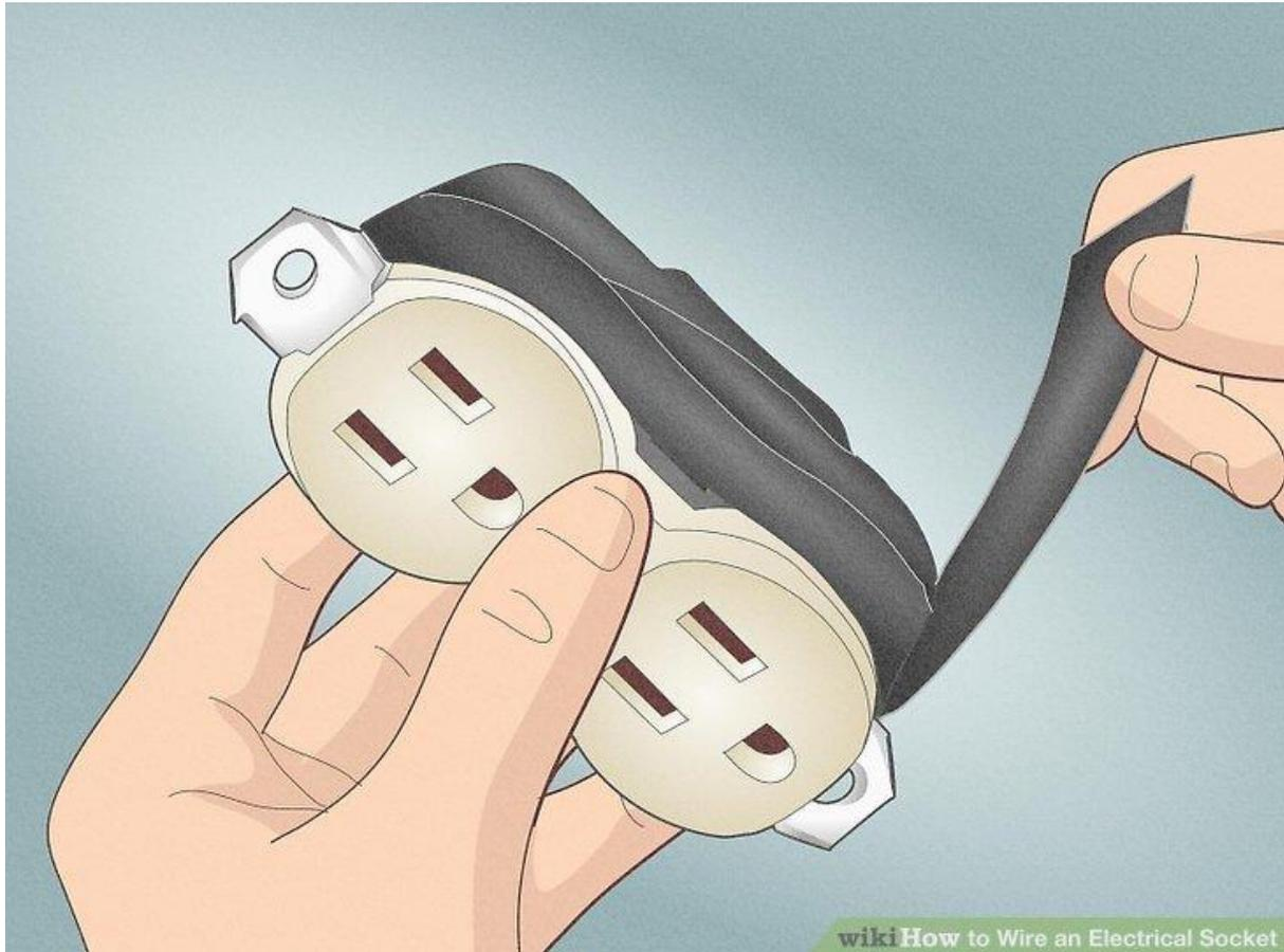
**Wrap the outlet in electrical tape.** For extra safety, wrap the sides of the outlet in electrical tape to reduce the chance of contact with a wire if it ever gets loose.<sup>[22]</sup> Your outlet is now ready to be inserted back into the wall.
