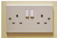
Sockets may be wired on [ring circuits](#) or radial circuits. Mostly rings are used, as they use less [copper](#) for most circuit layouts, they have [safety advantages](#) over radial circuits (sometimes debated), can provide more power, and cover more [floor](#) area per circuit.
